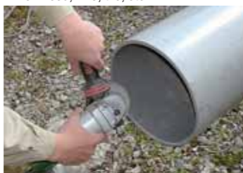
▲ Chamfering the inside edge of PVC pipe, etc.
